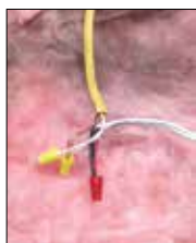
Open splice code violation!
