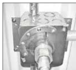
RUN CONDUIT IN TROUGH OR OVER RIDGE OF METAL DECK PAN
