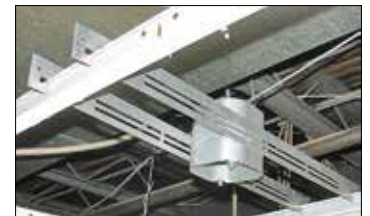
54181-TBAR IN USE ON DROP CEILING GRID
