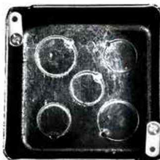
CONVERSION CLIP EARS INSTALLED ON OLD BOX
