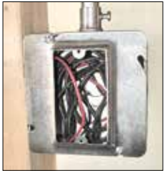
EXPOSED WIRES
