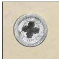
EZ ANCHOR INSTALLED
