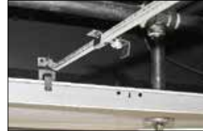
BHT1 IN USE ABOVE CEILING TILES
