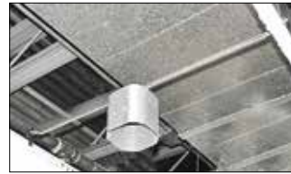
BHT1 IN USE ABOVE CEILING TILES
