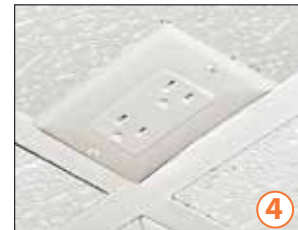
4 Cut ceiling tile and trim.
