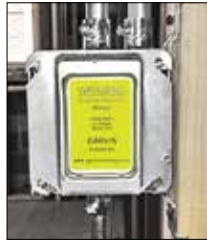
READY FOR DRYWALL
