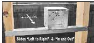
52181-ADJ IN USE Perfect position and adjustable depth to flush up with finished wall.
