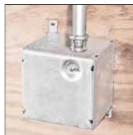
MOUNTED TO CONCRETE FORM
