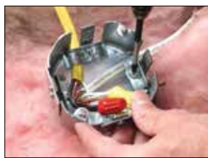
Secure cables with clamps.
