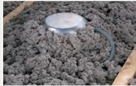
Insulated Ceiling (IC) type fixtures can be installed in direct contact with air permeable ceiling insulation. This allows the insulation layer to remain unbroken and prevent heating and air conditioning losses. These housings are also equipped with thermal protectors to guard against overlampping by cycling the lamp off and on until the problem is corrected.
