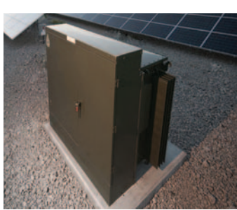
Medium voltage step-up transformer
