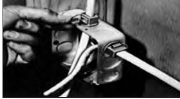
Snap captive locking wedge into connector's cavity.
