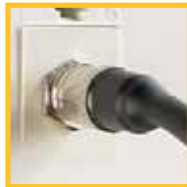
Trace Coax Cable
