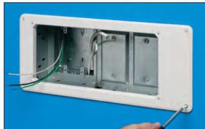
2 After drywall is installed, add trim plate, then install enclosure assembly to the wall with outer screws.
