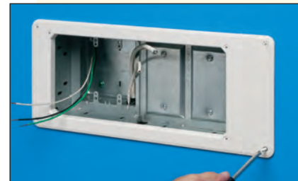
3 Install voltage separator.
