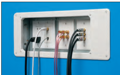
4 Install devices and plates.
