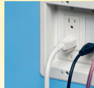
3 Install devices, then the wall plates.
