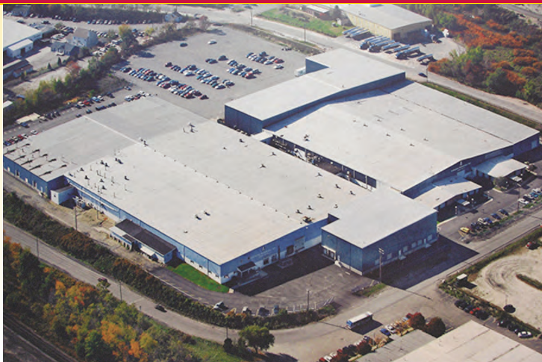
Arlington's manufacturing facility in Scranton, PA
