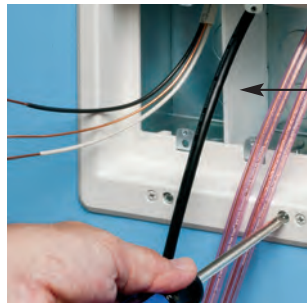
2 Pull cable. Insert box in hole. Tighten mounting wing screws to hold box securely against wall.
