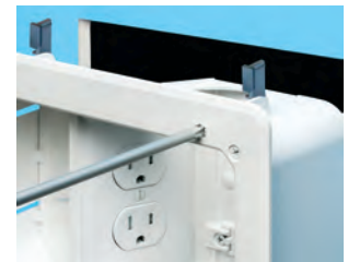
3 Place box in Top hole. Feed low voltage cables for TV through opening in box. Tighten mounting wing screws to secure box to wall.
