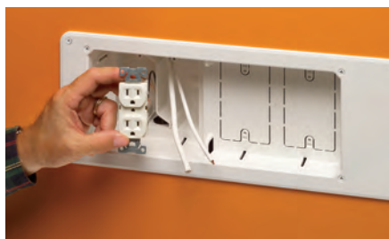
3 Install power and low voltage wiring devices.
