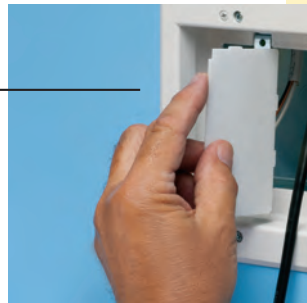
Note Install voltage separator for power and low voltage.
