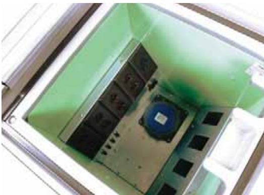
Convention Center Floor Box wiring compartment.
