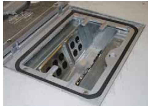
The interior of a CCBB Series Ball Room Floor Box.
