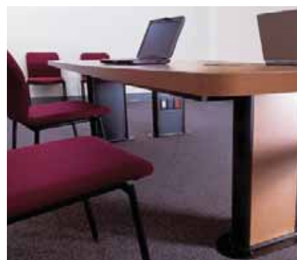
A Vista Point5 installation provides unobtrusive access to power and communication services in a conference room.
