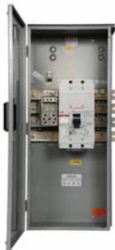
Main Circuit Breaker
