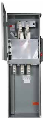
Main Fusible Switch with Utility Pull Box
