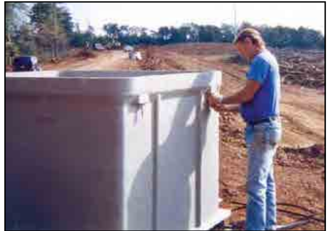
Attach nylon straps or chains to the lifting bolts (4.02).
