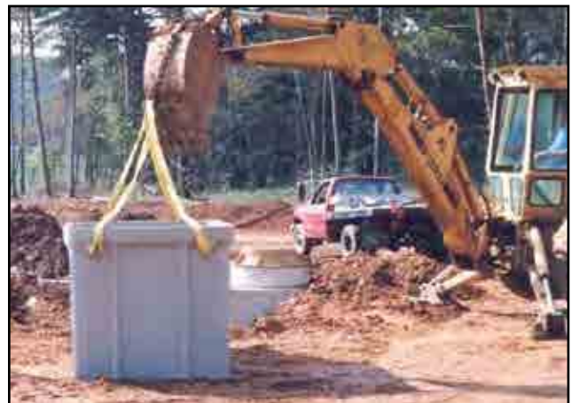
Lift and position enclosure with backhoe (4.03).
