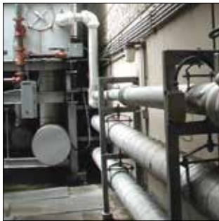
Pipe Freeze Protection
