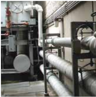
Pipe Freeze Protection
