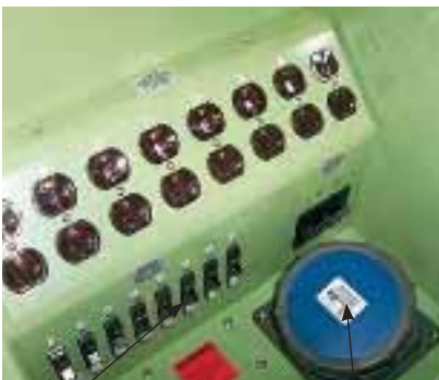
Circuit Breakers (Prewired to Receptacles)
