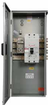
Main Circuit Breaker
