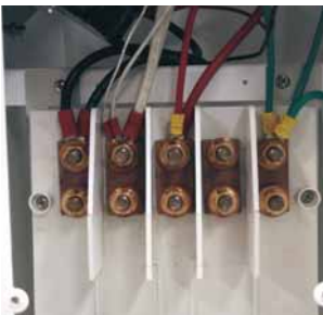
Copper Busbar with Ratings from 250 to 500 A
