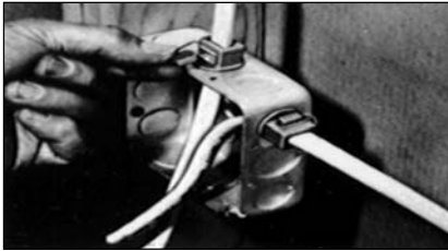
Snap captive locking wedge into connector's cavity.
