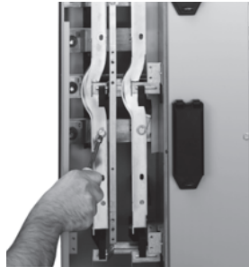
Field Phase Balancing
