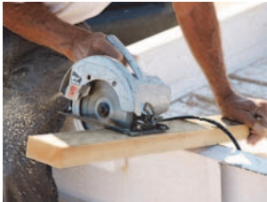
Construction Site Application
