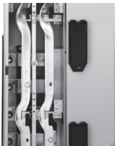
One-Piece Vertical Busbar
