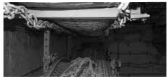
The systems after the fire-test
