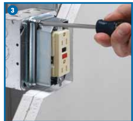
3 Re-tighten... Adjustment screws.
