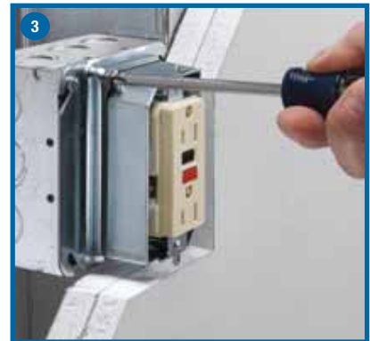
Re-tighten... Adjustment screws.
