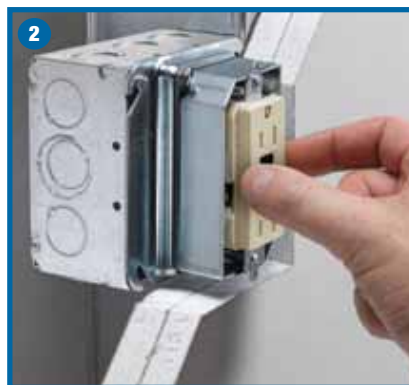
2 Adjust... Inner ring to be flush with wall surface.
