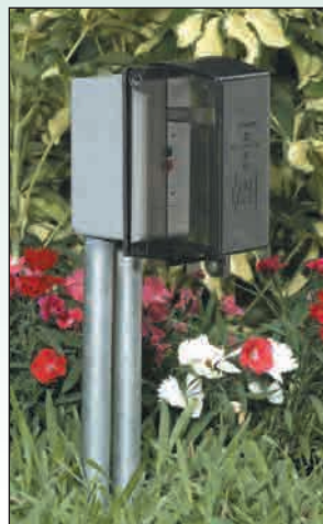
Why Install Boxes This Way...
