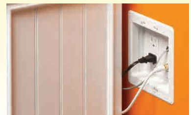
Finished Installed Shot.
