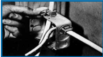
Snap captive locking wedge into connector's cavity.
