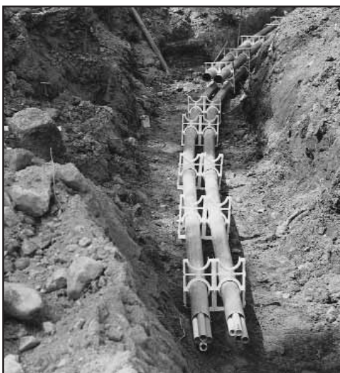
Pulled through existing conduits
