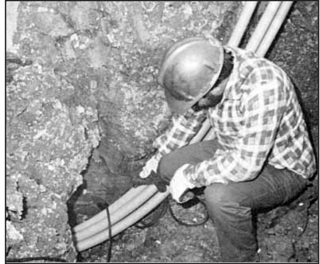
When soil conditions do not permit direct burial of cable, use Carlon P&C Flex® Nonmetallic Corrugated Conduit to protect the cable. A lower coefficient of friction provides easy wire pulls on location. flexibility eliminates the need for elbows.
