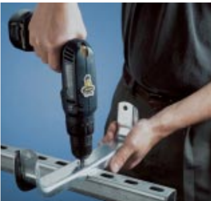
Mount U-Hook or Double J-Hook to strut.
