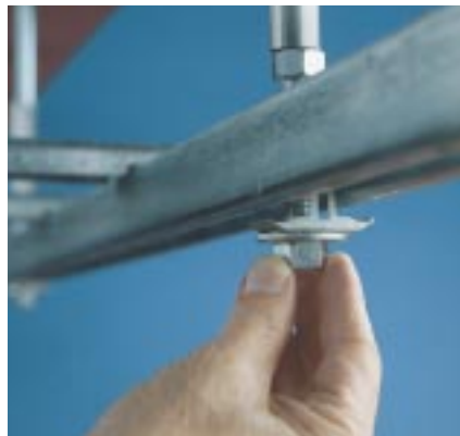
Mount strut to All-Thread Rod.
