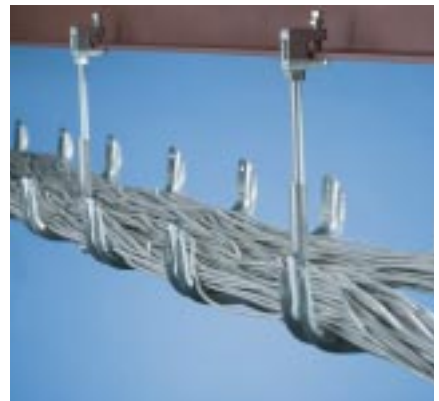
Mount assembly to beam.
