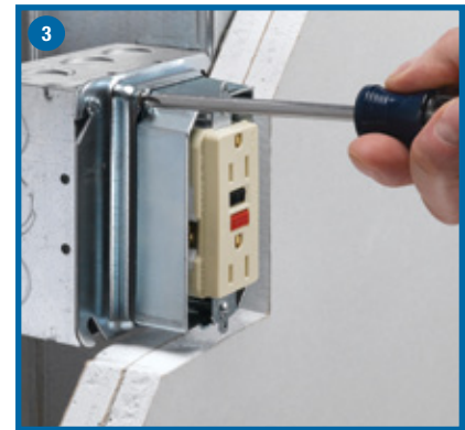
Re-tighten... Adjustment screws.
