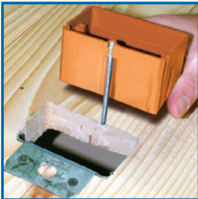
Install clip over subfloor.
