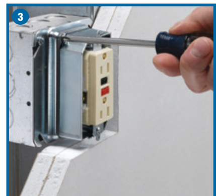
3 Re-tighten... Adjustment screws.
