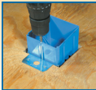
Screw in to adjust to height of flooring or carpet.
