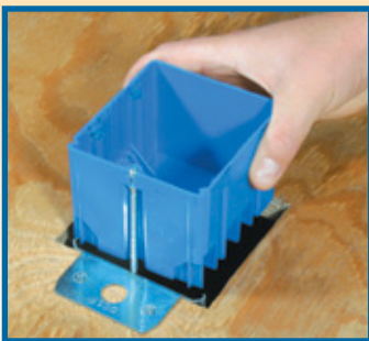
Install clip over subfloor.
