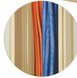
Route low-voltage cable
