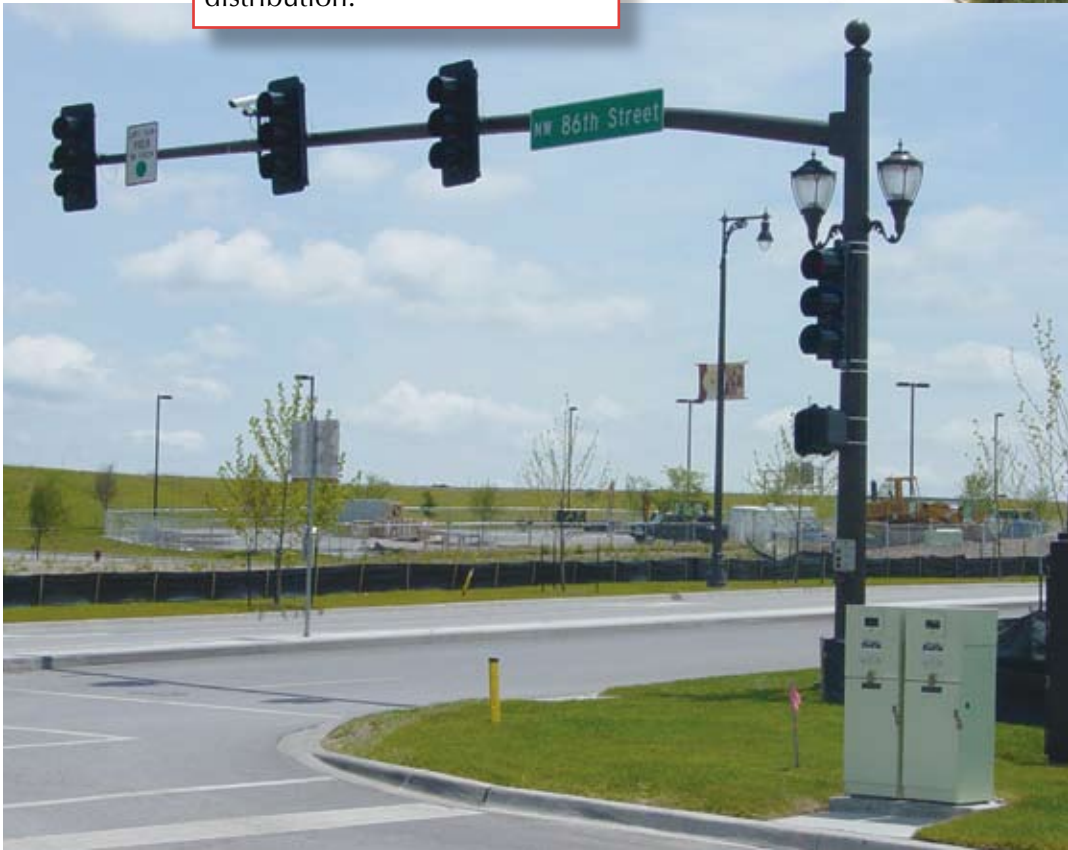
Location: Kansas City, MO Description: Zona Rosa Shopping Center. Multiple pedestal locations throughout shopping area providing street lighting and traffic signal distribution.
