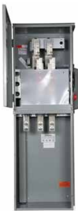
Main Fusible Switch with Utility Pull Box
