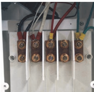
Copper Busbar with Ratings from 250 to 500 A
