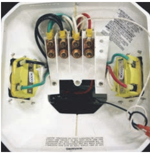
Copper Busbar with Ratings up to 140 A
