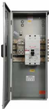
Main Circuit Breaker
