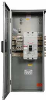
Main Circuit Breaker
