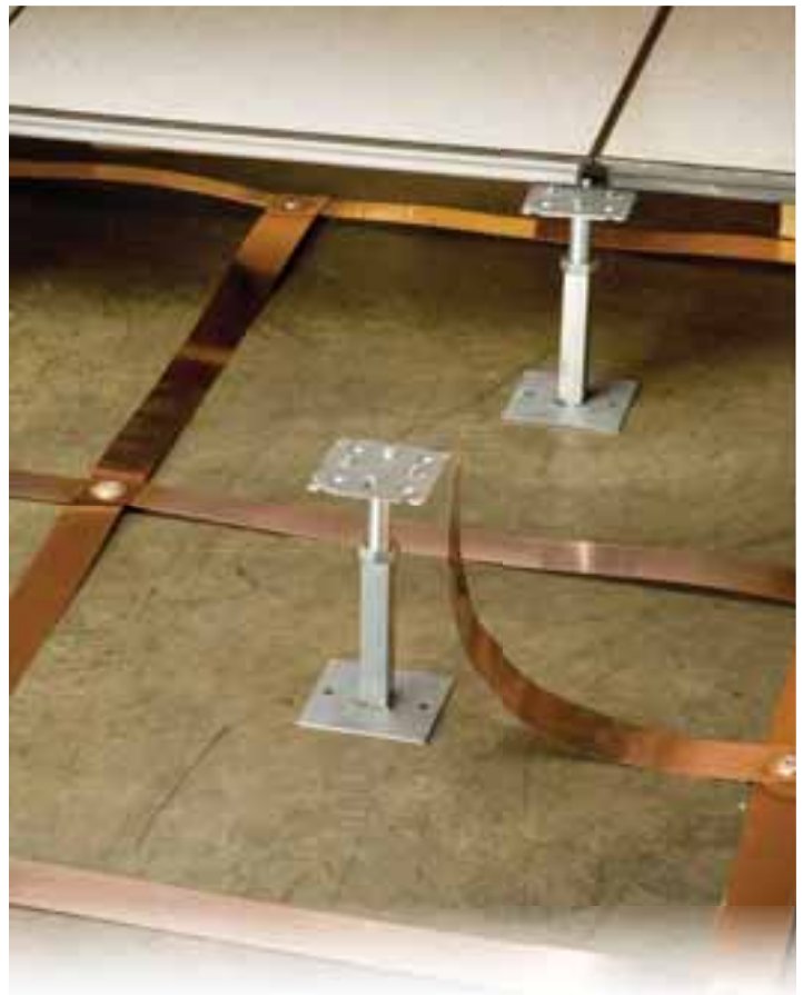
Pre-fabricated Signal Reference Grid installed under computer room floor.
