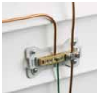
Intersystem Bonding Termination Bar (IBTB)
