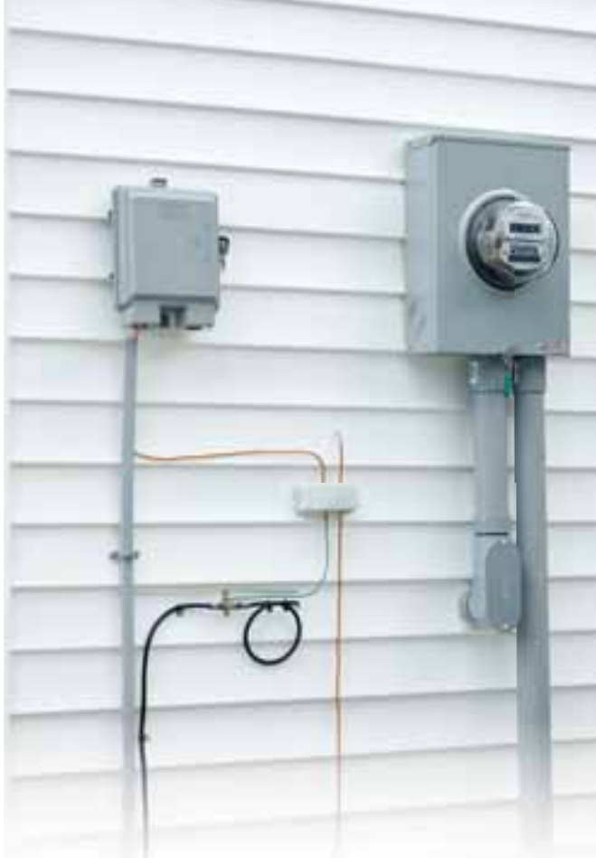
Intersystem Bonding Termination Bar (IBTB)
