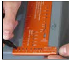
Step 1: Mark the first conduit.
