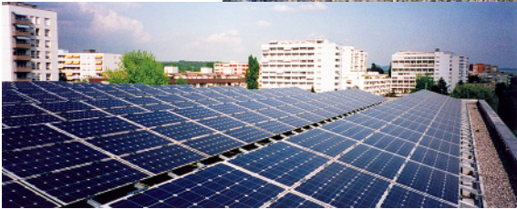
Photo: AS Engineering AG, Bern
