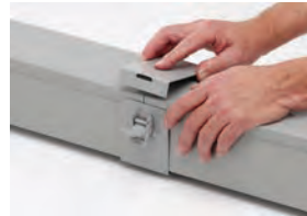
Install outside connector around wireway splice location
