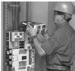
Panelboard Installation
