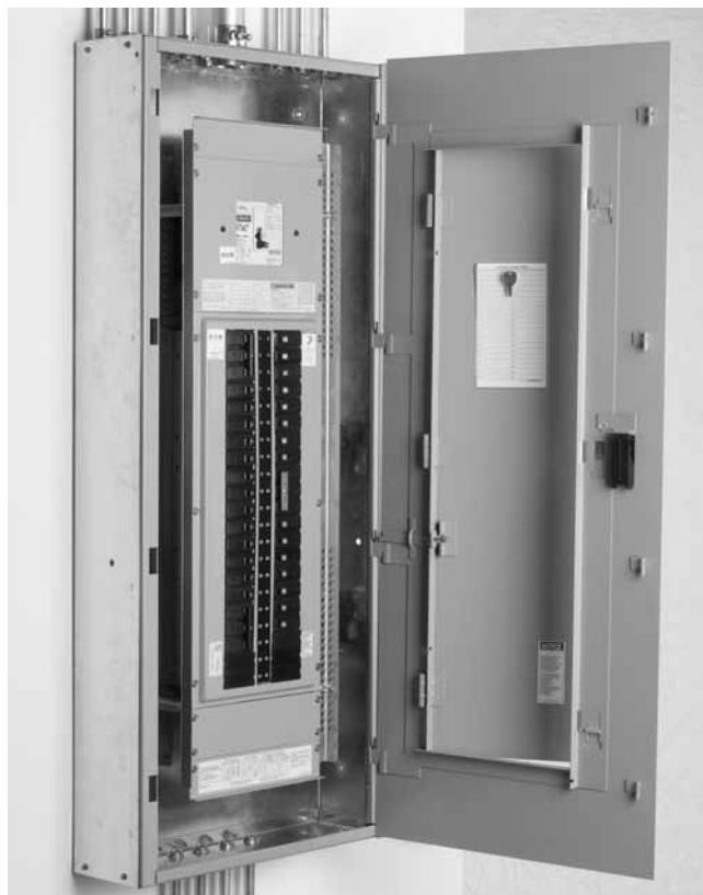
Trim Hanging on Surface Mounted Box
