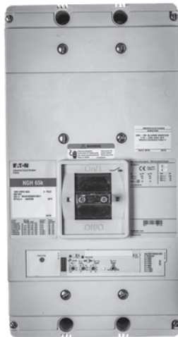
Electronic Trip Unit on SE Breaker
