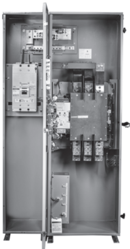
Separate Compartment for ATS and Breaker
