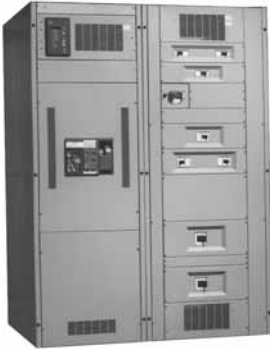
Front View—Circuit Breakers
