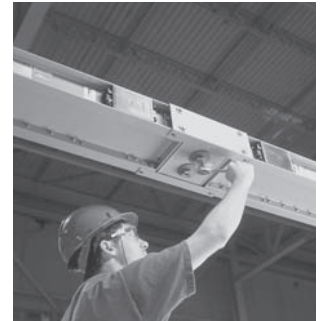
Typical Busway Installation (Torque Indicating Bolt)
