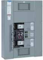
Elevator Control Panelboard
