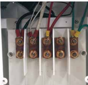
Copper Busbar with Ratings from 250 to 500 A
