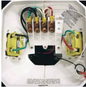
Copper Busbar with Ratings up to 140 A
