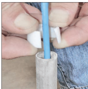
Snap on before or after cable pull.
