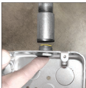
Insulated throat protects wires.
