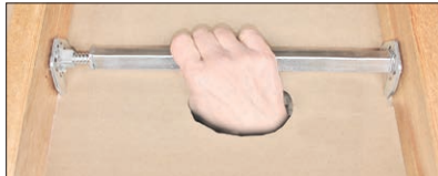
2) Twist out to bite on joists.
