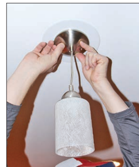
Wire & install new pendant fixture.
