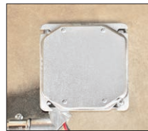
PROTECTED Ready for Drywall
