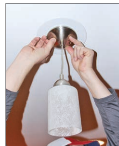
Wire & install pendant canopy.
