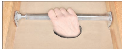
2) Twist out to bite on joists.
