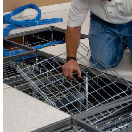
Place 2' tray sections in position.
