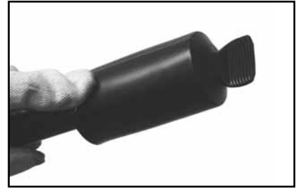
1. Slide the HSIC-FR end cap onto the cable and hold in place using forefinger or thumb.
