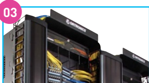
03 Mighty Mo Advanced Cable Management System with Clarity UTP Patch Panels and Patch Cords
