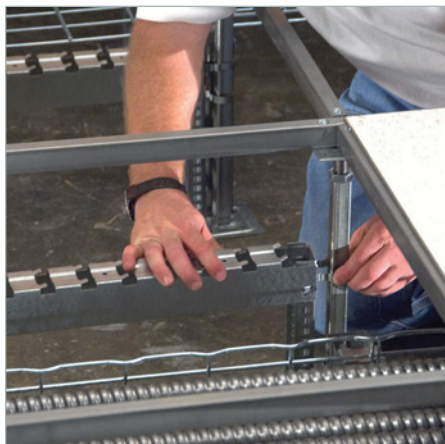
Supports and trays snap together without the need for complex tools or fasteners.
