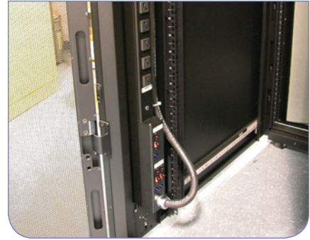
6B21N Power Commander Plus Power Distribution Unit shown mounted in an IT cabinet
