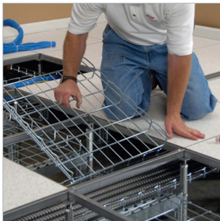
Tray sections are available in 2' lengths; 2", 4" and 6" depths; and 12", 16" and 20" widths.
