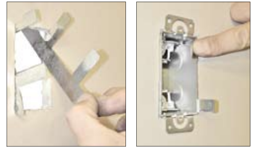
Insert supports. Bend support tabs.
