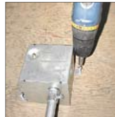
52181-SPKR IN USE On Concrete Form
