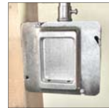
Wires are protected.
