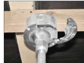
Hang pipe/ball assembly in cover, then connect wiring.
