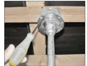
Secure cover with one screw.
