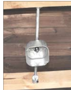
BH1 IN USE
