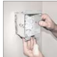
Cut hole, insert box
