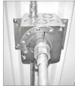
52181-DEK IN USE FOR HIGH-BAY LIGHT MOUNTING
