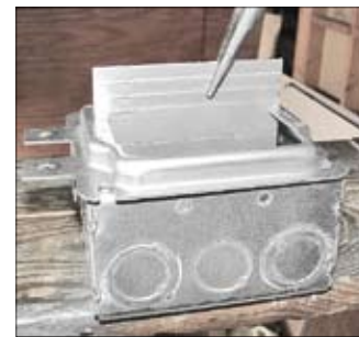
LVP42 INSTALLATION WITH BREAK-OFF TABS FOR EASY SIZING
