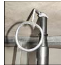
BR-400-SSC INSTALLATION WITH A POWDER GUN
