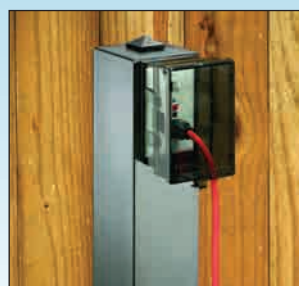
Finished with GFCI installation. (GFCI not included)
