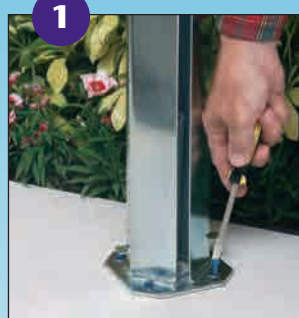
1 Metal support post attaches easily to surface.
