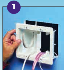
1 Using box as a template (without trim plate), mark location. Cut drywall. Attach trim plate to box. See Photo B. Install box assembly in opening.
