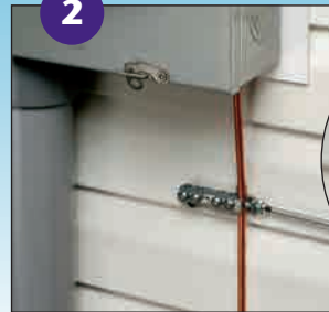
2 Insert grounding electrode conductor into the lay in lug. Tighten screw.
