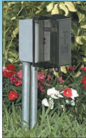
Why Install Boxes This Way...
