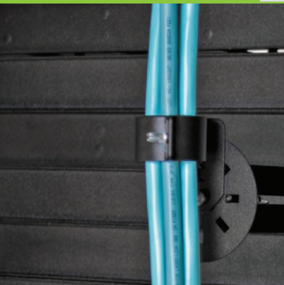
Rack-Mount Universal Clamp Kit Installed
