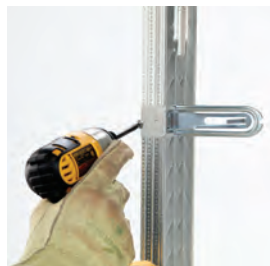
Support stays mounted to stud while securely attached with one screw
