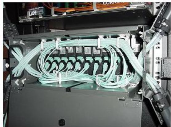
PCH-04U-EU-RH full equipped with 12 CCH LC-Duplex P&P Modules OM3 , integrated cable management
