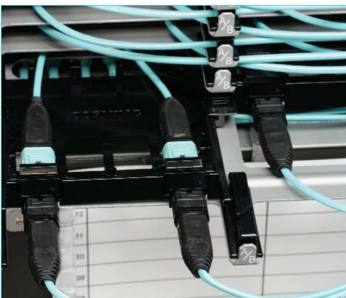
Pretium EDGE Solutions MTP Connector Panel Installed in Housing
