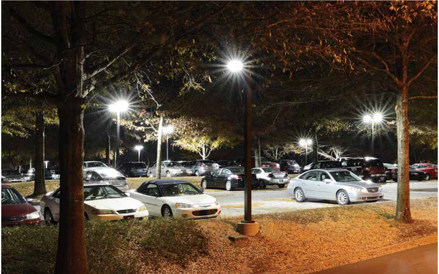
Kim Altitude™ installation at Clemson University, Clemson, SC
