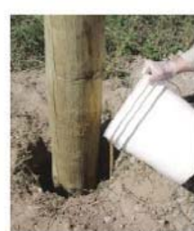
Pour mixture into prepared hole with pole
