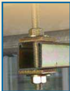
Standard method using nuts and washers.
