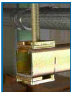
New method using Trapnut® Strut Fastener.
