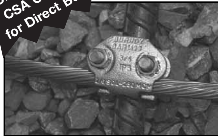
Wire to Rebar
