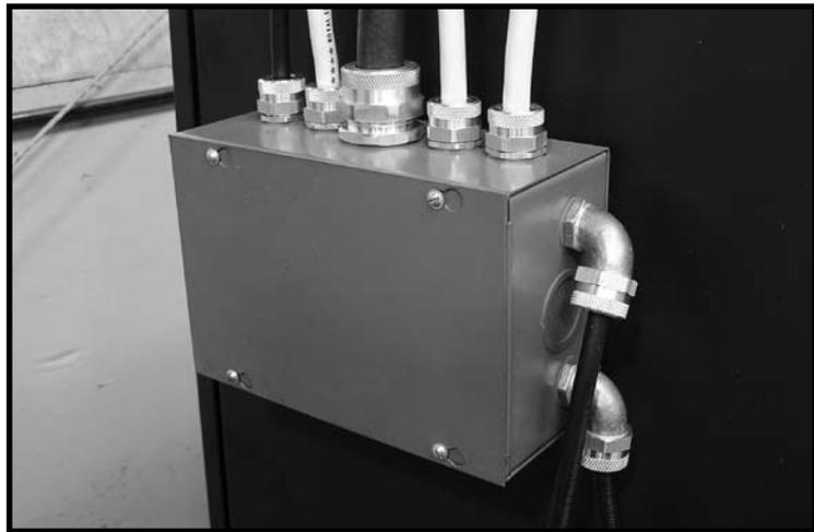
\*Cable jacket may have to be stripped to pass through connector.
