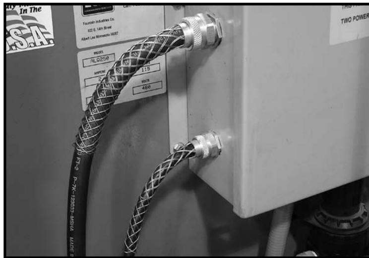
\*Cable jacket may have to be stripped to pass through connector.
