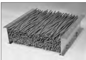
"50%" Fill Per NEC Cross Sectional Area Calculation
