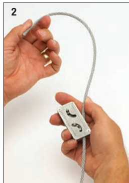
2 Loop wire rope through/around support
