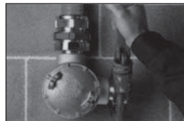
5. Install hub on enclosure
