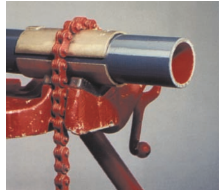
When a chain vise is used special care must be taken to prevent damage to the exterior coating.
