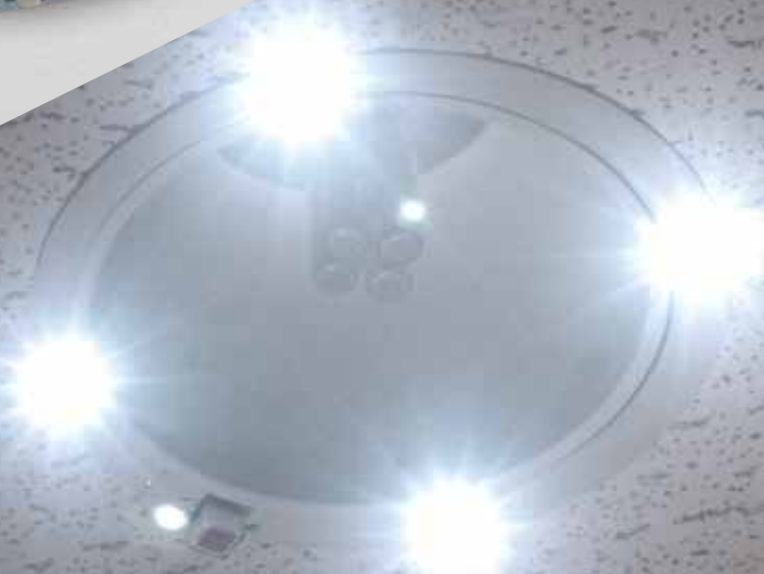
HOTSPOT1 IN OPERATION DURING POWER OUTAGE
