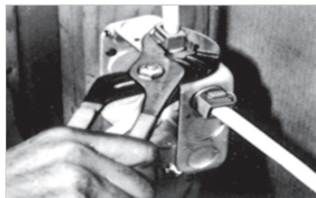
Press locking wedge into cavity which locks onto cable
